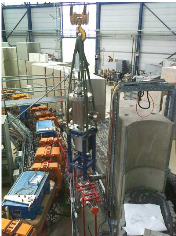
Fig. 1: Installation of the new beamshutter.
